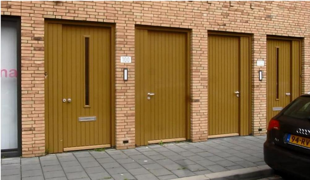
*Bicycle parking storage in a modern development in The Netherlands. The two doors in the middle open into bike storage rooms. Dutch building regulations require that residential cycle storage provides direct access on to a public road. The image below shows the internal layout.*
